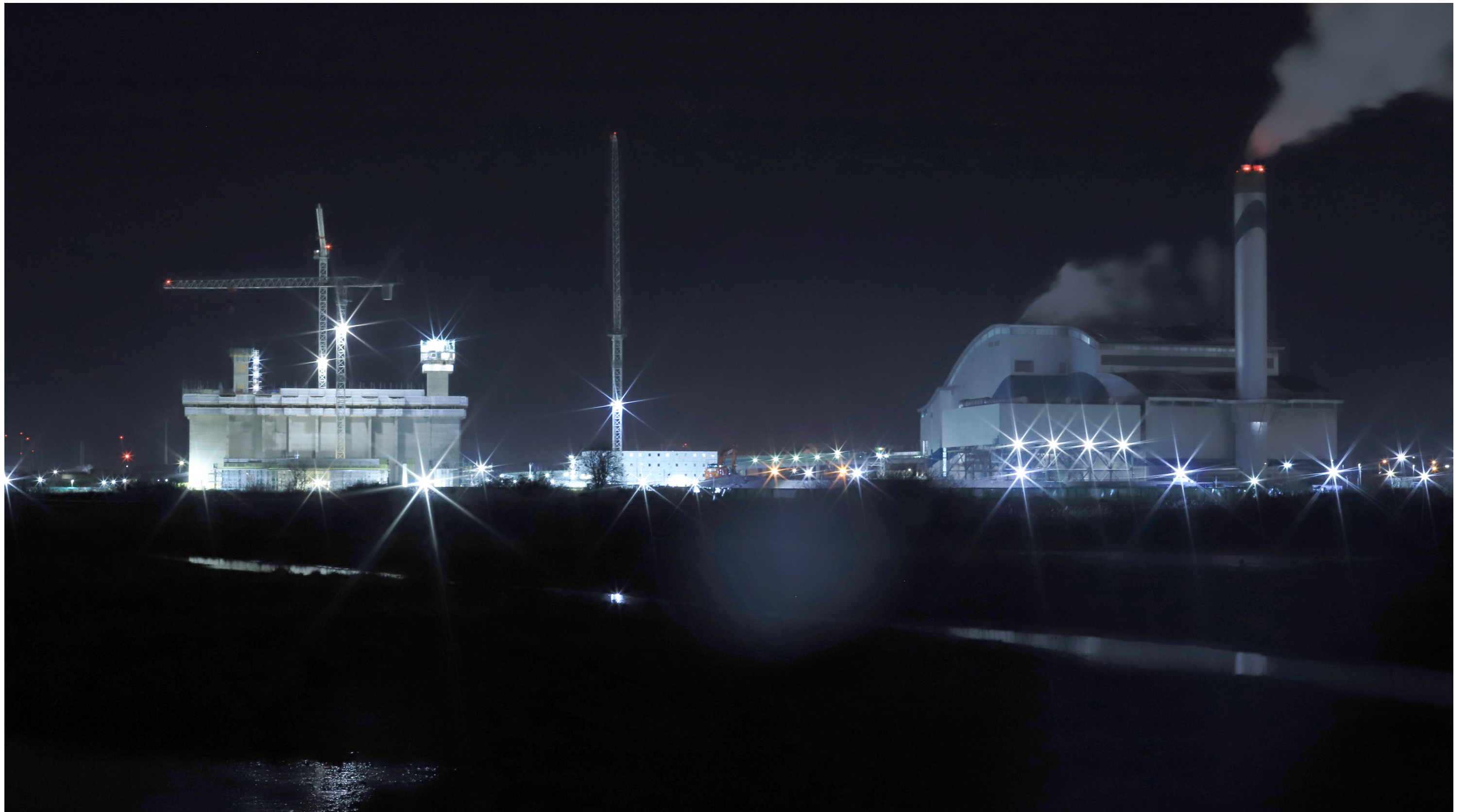
View 8: From Public Right of Way FP2, looking north
